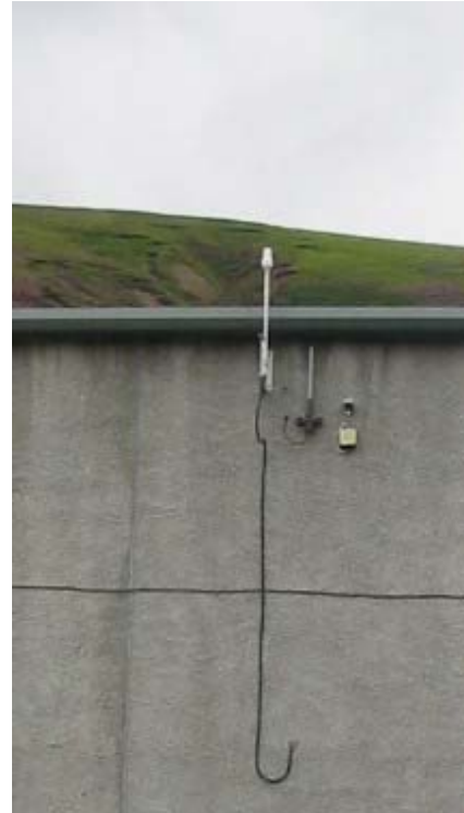
Water Reservoir Installation
