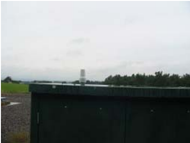
Equipment Cabinet Mounting
