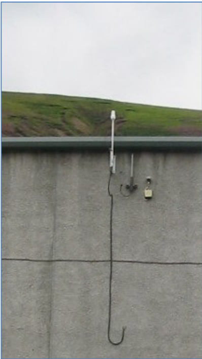
Water Reservoir Installation
