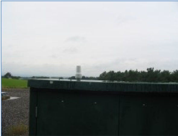
Equipment Cabinet Mounting
